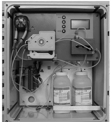
Figure 7: Completed pump tube installation
